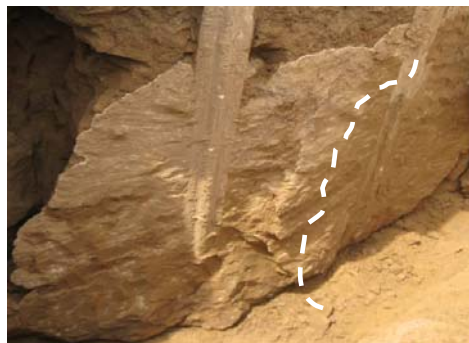
图4 高聚物劈裂注浆开挖效果 [16] Fig.4 Excavation effect of polymer grouting [16]
