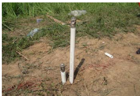
图2 现场安放注浆管 [16] Fig.2 Grouting tube after placing [16]
