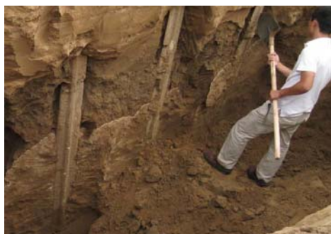
图3 现场开挖 [16] Fig.3 Site excavation [16]
